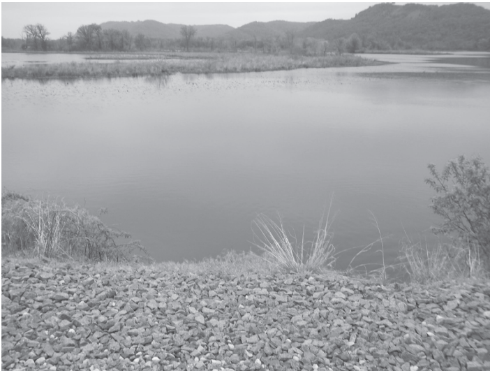
Figure 1. View from the northwest side of culvert.
