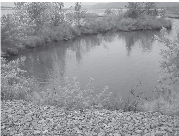
Figure 2. View from the southeast side of culvert.
