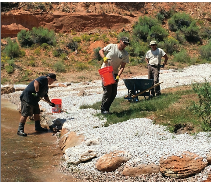
Hardening the streambed at the crossing required heavy equipment and a great deal of hard, physical labor (left column), but the final result (right) will benefit local residents, both human and aquatic. (Photos by USFWS)
