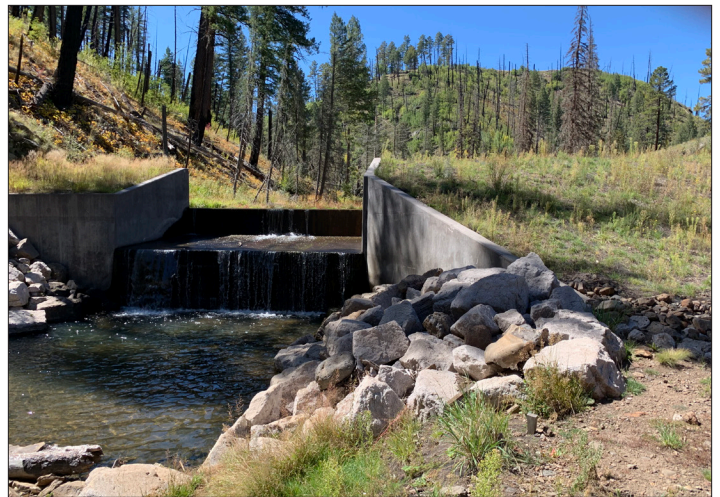
Figure 10. The barrier dam on Willow Creek that prevents non-native trout from recolonizing upstream.
