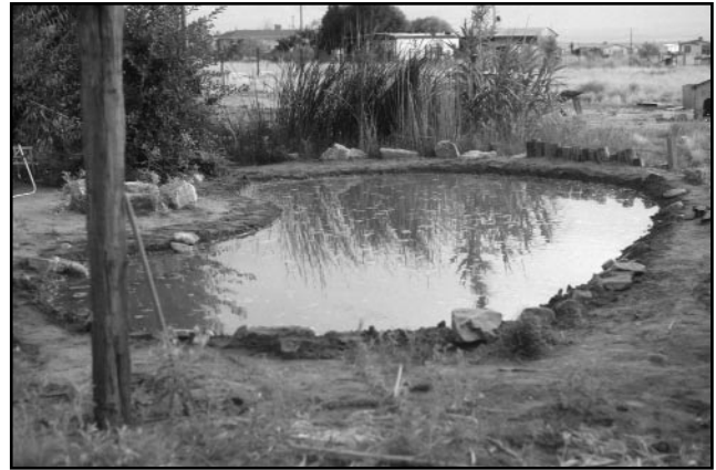
Fig. 4. Hiding the liner. should be chemically inert unless your goal is to keep hard- or brackish-water species.
