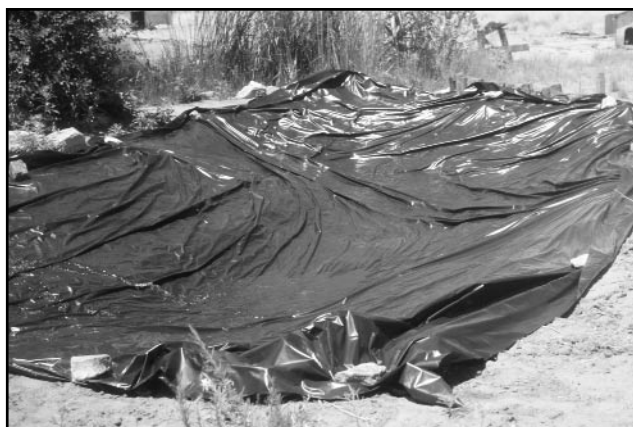
Fig. 2. Laying the liner.
