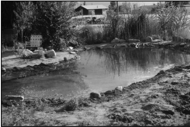
Fig. 3. Covering the liner and adding stone.
