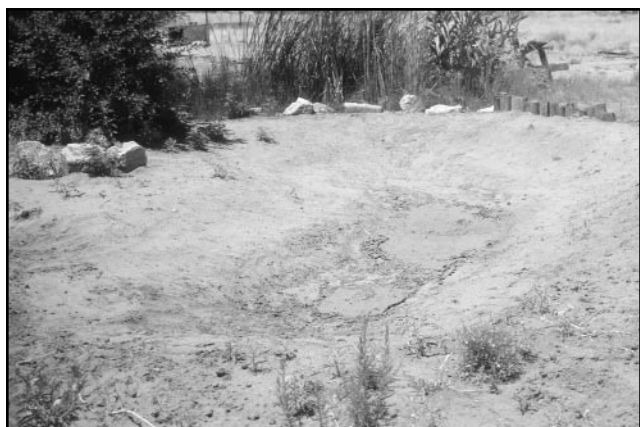
Fig. 1. The hole before laying the liner in place.
