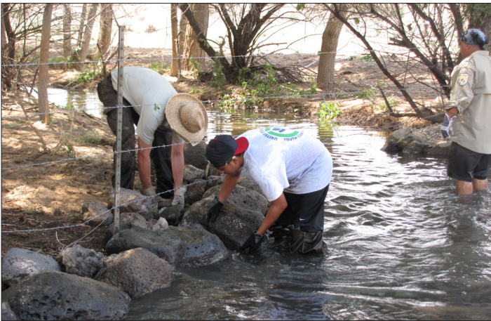
Xavier Lovato and NMFWCO staff member Jason Davis position rocks to stabilize the bank of the lower Santa Fe River.
