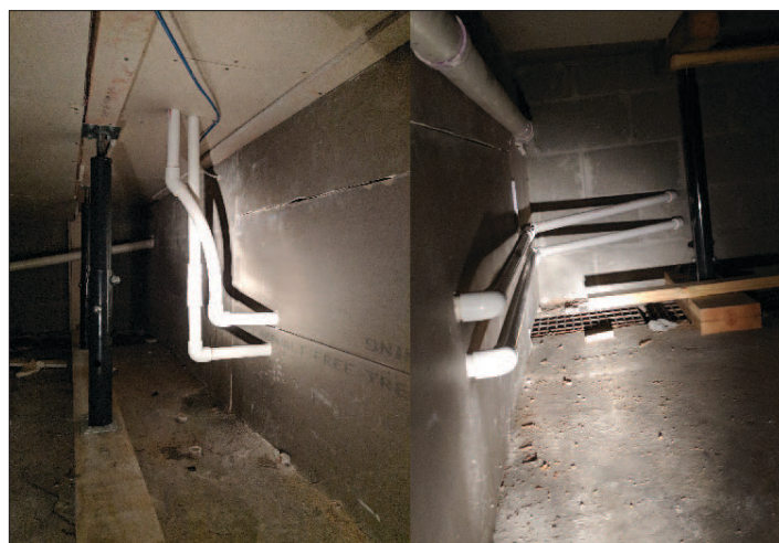
Figure 3. Convoluted plumbing in the basement.
